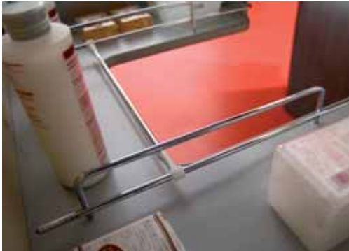
Drawer accessories for basin unit allowing waste and bottle trap accommodation.
